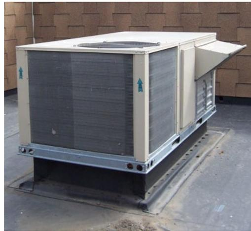
**Figure 5. Packaged Air Source - Air Heating/Cooling Heat Pump**
