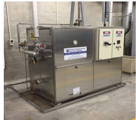
Figure 2. A modern compact electrode steam generator
