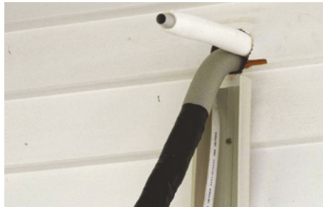
Figure 7.19 Bind insulation with vinyl tape
