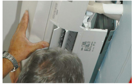
Figure 7.10 Attach unit to wall bracket (B)
