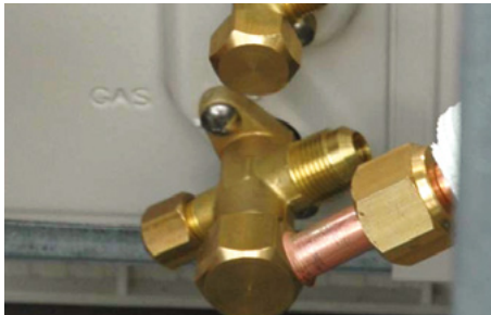
Figure 7.27 Connect pipes and tighten flare nut
