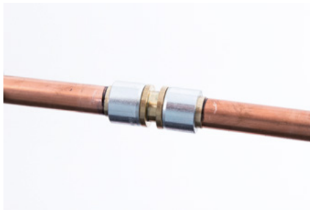
Figure 6.10 Step 9: Completed compression connection
