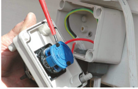
Figure 9.4 Install lockable isolating switch (C)
