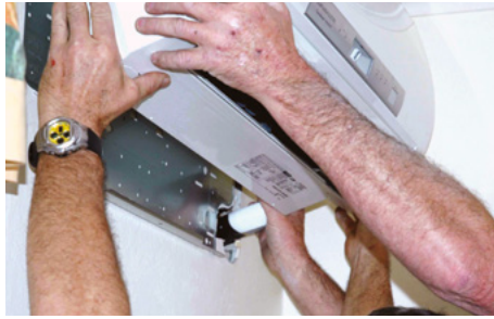
Figure 7.9 Attach unit to wall bracket (A)
