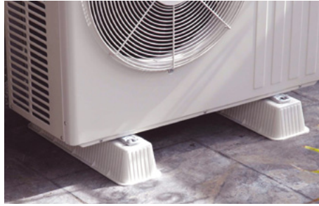
Figure 7.14 Unobstructed gap under outdoor unit fixed on concrete pad cast in place
