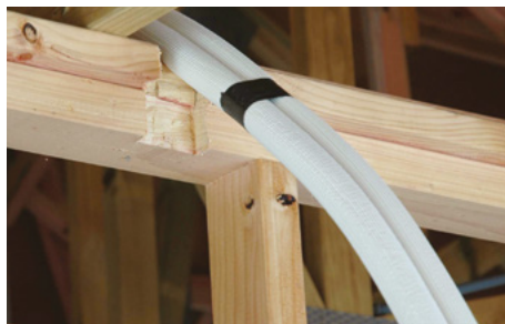
Figure 6.27 Notch the top plate and studs (A)
