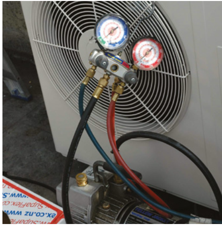
Figure 7.31 Remove vacuum pump and gauges (C)
