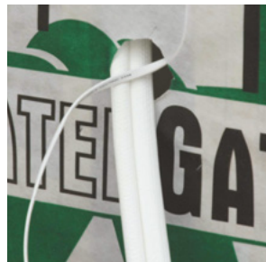
Figure 6.33 Feed pipe/cables through building wrap
