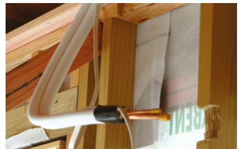
Figure 6.28 Notch the top plate and studs (B)
