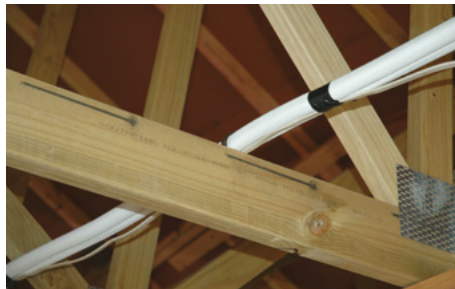
Figure 6.26 Run pipe/cable across truss chord/ceiling joist
