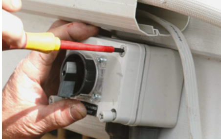
Figure 9.4 Install lockable isolating switch (C)
