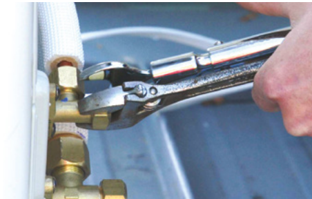
Figure 7.28 Tighten flare nut connections
