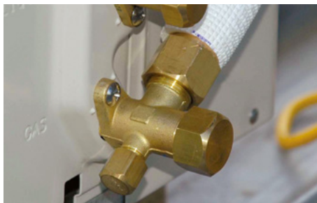
Figure 7.33 Tighten valve caps
