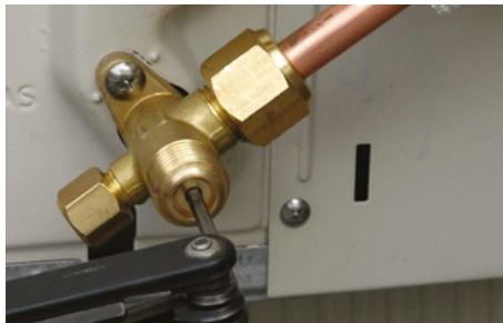
Figure 7.32 Progressively release the vacuum
