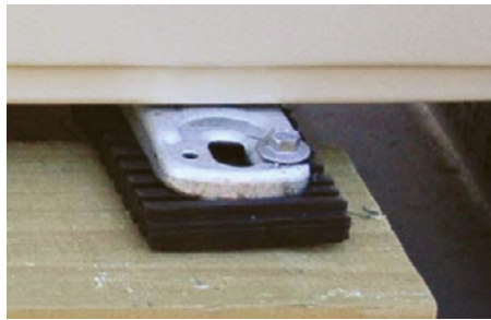
Figure 7.17 Pack with plastic shims to level
