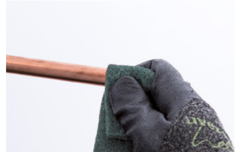
Figure 6.3 Step 2: Roughing the end surface
