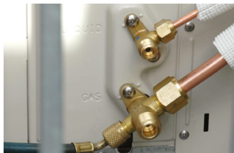
Figure 7.29 Remove vacuum pump and gauges (A)
