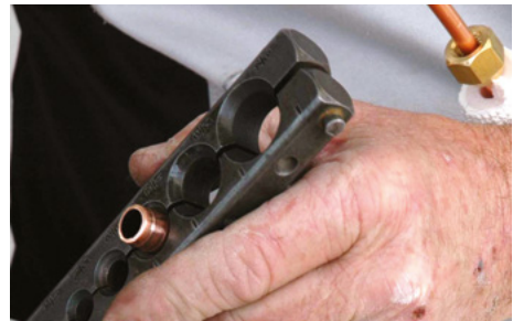
Figure 6.17 Flare the end of the tube (A)
