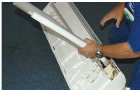
Figure 7.5 Release the tubing and drainage hose
