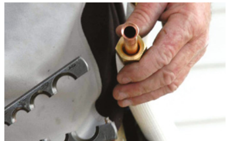
Figure 6.19 Flare the end of the tube (C)
