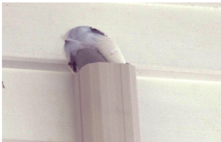
Figure 7.23 Fill hole around piping with sealant
