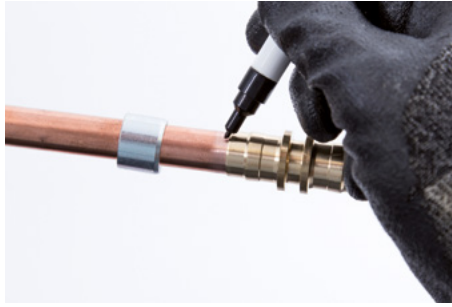
Figure 6.6 Step 5: Fitting connector marking stopline
