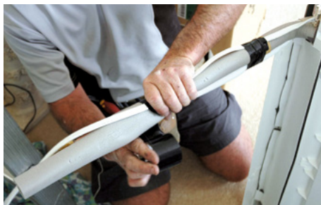
Figure 7.7 Tape tubing, drainage pipe and connecting cable together
