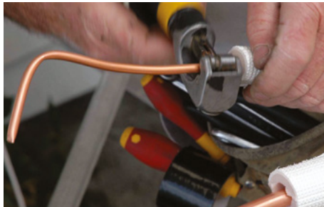
Figure 6.14 Cut pipe with tube cutters
