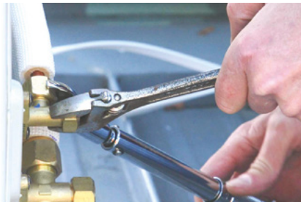
Figure 6.24 Tighten connection (A)
