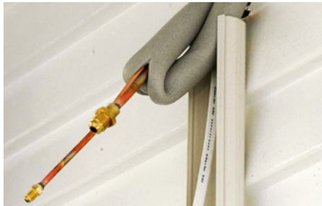
Figure 7.13 Expose flared pipe ends
