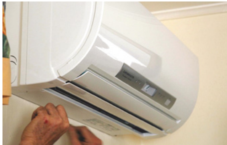
Figure 7.11 Ensure unit is securely seated
