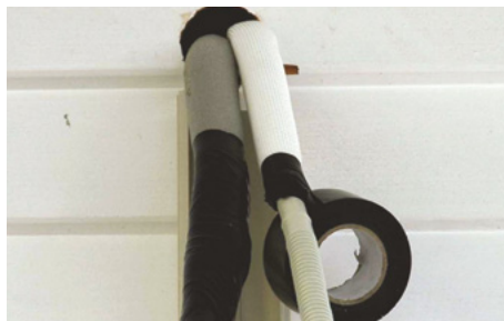
Figure 7.20 Tape drainage hose to drainage outlet
