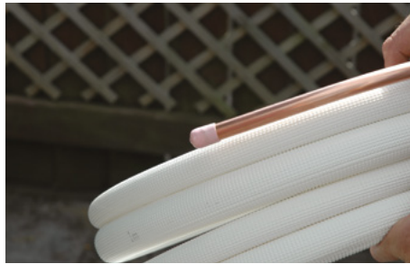
Figure 6.12 Cover pipe ends
