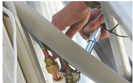
Figure 6.25 Tighten connection (B)
