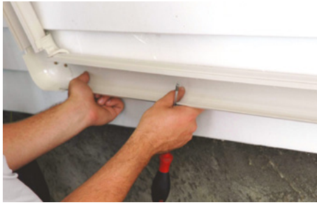
Figure 7.21 Install trunking neatly
