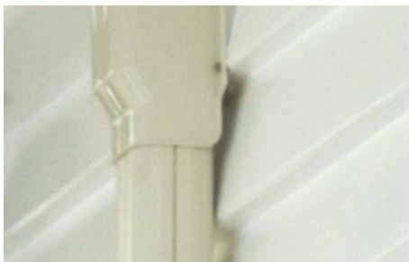
Figure 7.25 Fit cover over opening
