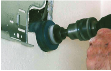
Figure 7.3 Drill a hole through the wall
