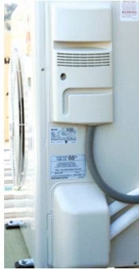
Figure 9.5 Replace service cover to outdoor unit
