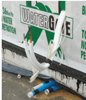
Figure 4.10 Pre-install pipework before building claddings are installed
