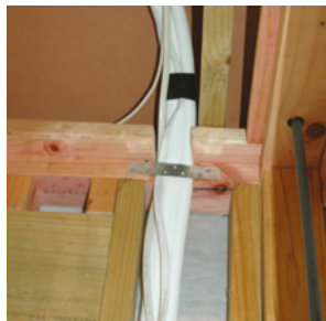
Figure 6.32 Fix galvanised mild steel strap to hold pipe/connection cable
