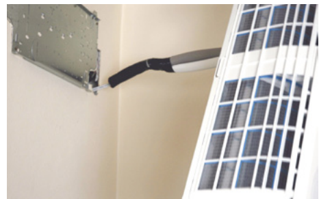
Figure 7.8 Feed taped bundle through the hole
